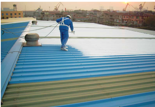
Build Bond 1K/SB apply on Metal Roof
