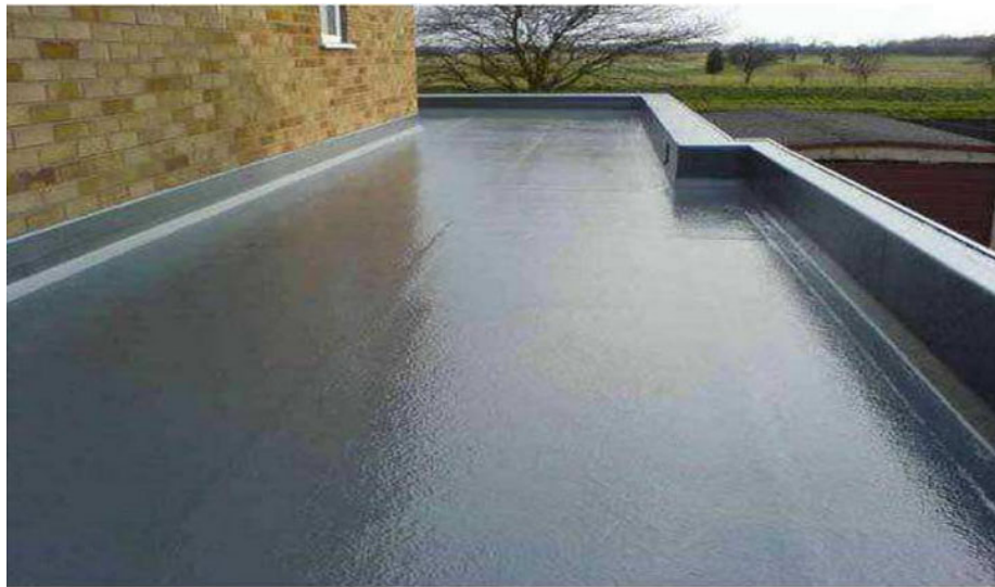
Build Bond 1K/SB apply on R. C. Roof
