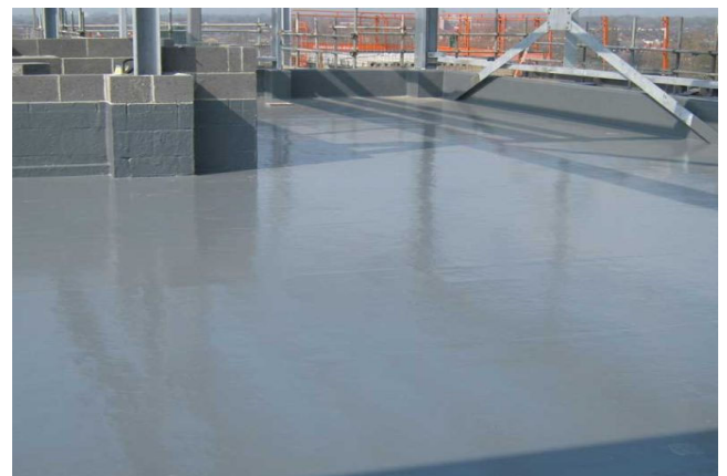
Build Bond 1K/SB apply on R. C. Roof
